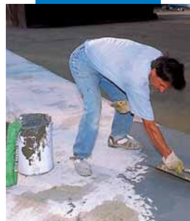
Hydroizolace bazénu Mapelasticem
